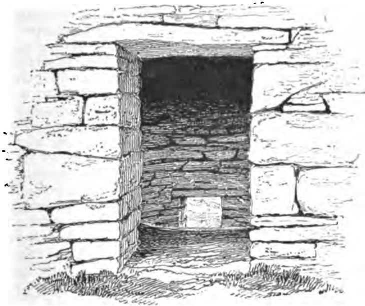
Fig. 9.—Ope of Low Entrance. No. 2. Taken from Interior of Cashel.
